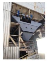
Bristol Concrete Plant has recently had a new aggregate weigh hopper fabricated and fit by Response Engineering. This meant that the Plant was on a week's downtime once they returned to work in 2016.
