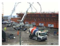
Congratulations to everyone working on the new Mersey Gateway project. Work has started on the approach viaduct decks, with the first continuous 34 hour pour of 1,148m<sup>3</sup> concrete using 12 trucks having just taken place.
