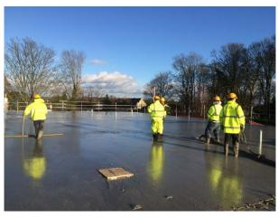
Last week CEMEX Croydon Plant became the first in the country to produce a new branded mix called Advanced Decking. Advanced Decking is a selfcompacting, self-levelling flooring concrete for floors in modular buildings and was designed in partnership with Propex.
