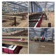
Coventry plant has successfully supplied 180m3 of Evolution Structural to the new London Taxi Company assembly plant in Coventry. The concrete was used to fill the underneath of a metal frame conveyor belt. The factory will be used to build the next generation of electric and low emission vehicles.
