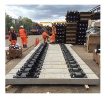
A little over 12 months ago CEMEX Rail Solutions were asked to attend a meeting with London Underground. This was to help them come up with a design of concrete bearer for curves of less than 200m radius. The particular issue with tight curves is that of wheel / rail alignment around the curve. The way to ensure that wheels remain on the track is by use of a check rail next to the running rail; this guides the wheel and keeps it on the rail.
