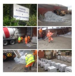
Cannock Readymix Plant was on hand to supply a local aluminium casting factory with MicroTech concrete for its high early strength and abrasion resistance properties. Norton Aluminium and Casting Ltd have requested a fast setting concrete that would cure within 6 days, with the extra properties to withstand the challenges faced. The concrete supplied has been used to repair the storage bays for the freshly processed recycled metals.
