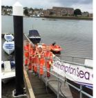
Planning the work was not simple as access to the jetty piles was only possible over low tide, so the Team was split in to 3 groups who worked on 3 separate days over the 5 hour low tide period. The work was completed on August 12th with all 3 piles having had 2 coats of paint.
