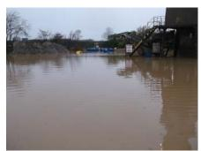
The picture shows Brunswick (near Newcastle upon Tyne) concrete Plant after the recent heavy rain. The yard was flooded due to a surface water drain being blocked by a farmer carrying out drainage work in the field adjacent to the Plant.
