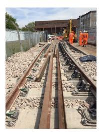
London Underground recently won the award for Track Technology at the UK Rail Industry Awards for their concrete check rail bearer which was developed jointly with CEMEX Rail Solutions.
