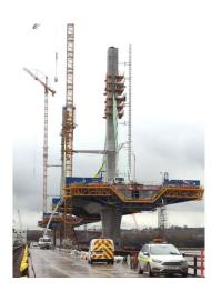
An impressive Mersey Gateway shot as they start the 120m3 concrete pour for a deck segment on the Central pylon.
