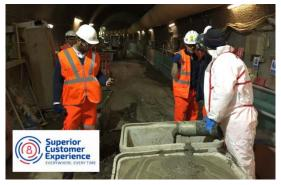
A successful site trial was carried out for FLO JV at Kennington for the secondary lining to the Northern Line extension in London. The mix was pumped 50m down and 250m horizontally; the mix needed to reach consistence retention in four hours.
