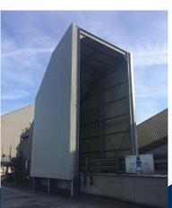
Tilbury has invested in installing two tipping frames over the apron belt feeders to ensure the safety of drivers and others should a vehicle tip over.
