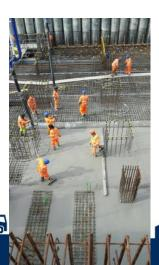
Last Tuesday CEMEX Readymix Area 20 completed a 650m3 pour for John Graham Construction for the new Energy from Waste Plant in Gloucestershire. The pour was comprised of 2 mixes, a C45 DC4 and a C45 DC4 Caltite. CEMEX had to dual supply both mixes to two different pumps from three different plants and with a 4am start - the challenge was set.
