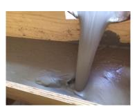
Matt Doran reported that Berkswell Readymix Plant successfully produced its first ever POROFOAM 950 for Costain Ltd, working at Claverdon Sewage Treatment Works in Warwickshire. The customer was looking for a non-structural mix to fill an underground chamber.
