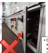
Defective isolator handle allowing access to panel with isolators "closed" or "open and locked out"
