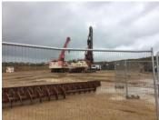
The drilling rig and crane arrived at Denge Quarry recently ready to start drilling and sheet piling for the new shoebox berth. This is the first stage of the new berth being constructed at Denge Quarry. Once constructed the site will have a new way of working which will be with a 360 excavator on a pontoon working over the water - this will give the Quarry an extra 8 to 10 years of life.
