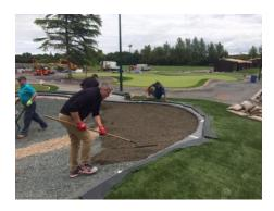
Back at the start of the month an enquiry was made for 6m of 'Capillary' concrete from a company called Border Sports Services - a national sports turf specialist based in Carlisle. The customer was looking for a permeable concrete with a very specific mix design and voids percentage, for use as a sub-base in a golf bunker. The customer then wanted to add their own Capillary Admixture to help draw moisture from above (when the ground was too wet) as well as from below (when it was too dry).
