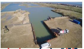
The life of Denge Quarry is being extended by 8-10 years thanks to an excavator on a pontoon allowing us to excavate to the maximum depth for sand and gravel. Six mooring bollards have been fabricated and installed.
