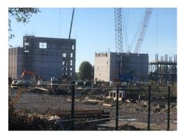
A couple of months ago we saw the successful pour of the above ground Slipform for Grahams Construction, Javelin Park Gloucester. Over the last week there seem to be a new arrival in the Slipform family, a duplication of the first one but at a smaller scale.
