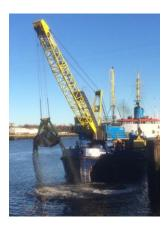
The team at Jarrow Wharf has the Cherry Sand from UK Dredging on site for a second visit in an attempt to remove materials that have accumulated over the years due to a stand off from stumps left when the original wharf was demolished.
