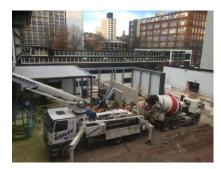
The Readymix North West team supplied a Steel Fibre Concrete pour for expanded structures at Project GEIC Manchester. The project, in both a commercial and residential area, required a solution to provide a high quality finish.
