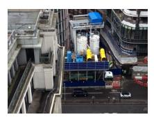
The site is located directly on London Bridge! – It is very difficult to access and a special lane separates pedestrians and other vulnerable road users away from site traffic. Each silo holds up to 100 tonnes of dried sprayed concrete blown in by the road tanker.
