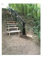
concreted-in posts to stabilise the hand rail and repainted it, offering it a few more years of use.
