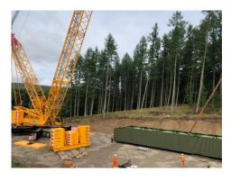
Cambusmore Quarry has finished installing their new conveyor bridge across the river Teith. The bridge has been installed so that the Quarry could access new reserves on the west bank of the river. The only other option was a large detour north through a country town called Callander.
