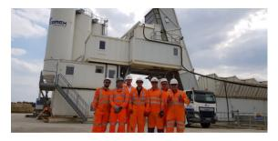
As CEMEX and home counties Readymix prepare to open our latest Readymix plant at Bramshill quarry, the LIEBHERR 2.25 mobile mix plant is a true reflection on the investment that CEMEX is making within the UK. The plant is to replace the existing Eversley Readymix plant which has produced concrete for many years.
