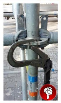
The injured person is an employee of a subcontractor for scaffolding works. Together with two more colleagues, he was dismantling a scaffolding at a clinker cooler building; there were no lateral guard rails and toe boards at the time of the incident.
