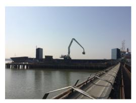
The installation of the new hopper on the jetty is nearing completion. This will give all of the CEMEX Marine dredgers the capability of discharging material into Dagenham Wharf.
