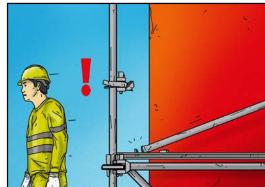
Any damage to the scaffolding must be reported. Do not remove any scaffolding parts.
