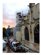
After the terrible fire that devastated Notre-Dame last April, CEMEX is participating in the preparatory works for its future restoration. From its Paris-Ivry site, CEMEX supplies several formulas of ready-mix concretes, including highperformance concretes, for the slab built by the construction firm BJF. This technical work will encapsulate the first floor of the crane that will cover the surface of the damaged structure of the building.
