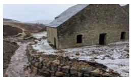
Leyburn recently supplied rock armour to a riverbank reinforcement project - this project in Swaledale aimed to rescue a disused Smelt Mill at risk of collapse due to last years' flooding.
