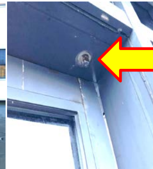
Location of where door dropped from frame pin
