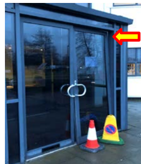
Location of where door dropped from frame pin
