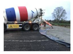
This week the team delivered 400m3 of CEMEX Advanced Paving out of Northampton with the help of the Bletchley plant. This is a VAP product that has saved the customer time and effort as it has replaced the need of using steel mesh. By midday they had supplied 335m3 which enabled the customer to finish at a reasonable hour.
