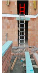
The access ladder in unsatisfactory technical condition
