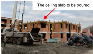
The ceiling slab to be poured
