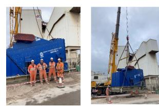
The team at Salford Asphalt plant are very happy to receive the investment in a new screen on site. It represents a large investment in the plant and is a state-ofthe-art water cooled screen designed to increase the life of the bearings, reduce servicing and therefore downtime.
