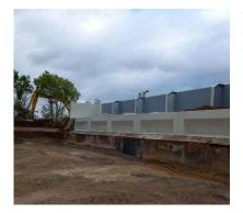
The team at Salford asphalt have installed seven new cold feed bins to replace the 40 year old units that were in place. The cold feed bins hold aggregate that is used in the asphalt production process.
