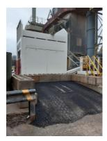
Great to see the latest Health & Safety improvement made at the Preston Asphalt plant – a ramp has been constructed using concrete lego blocks and asphalt to give better/safer access for loading of the new RAP bin.
