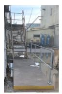
As part of ongoing 5S activities at Salford Aggregates & Asphalt plant, a new raised walkway has been added to prevent site ponding in various areas, which previously happened because of historical badly designed raising of road ways.
