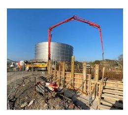
The team from our Blackburn Readymix plant recently supplied our key customer, Stem Construction, with over 300m3 of Readymix concrete. This was for the base of the second storm tank at Rossendale Waste Water Treatment Works.
