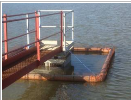
Before Original Weir Box
