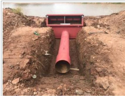
Base of Weir Box
