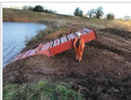
Weir Box following embankment.
