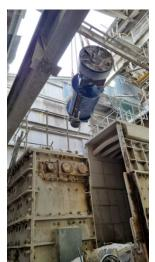
Over the Easter Bank Holiday weekend the team at Dove Holes quarry undertook a massive investment project to replace the 26 tonne rotor using 500 tonne crane.
