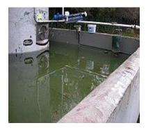
Effective bunds will collect and contain anything which falls inside them, not only the liquid they are designed to capture but also unwanted material such as rainwater. If a bund is not maintained properly the unwanted build-up could reduce the capacity of the bund and may cause it to fall below the capacity requirements. Rainwater and other debris should be removed regularly.
