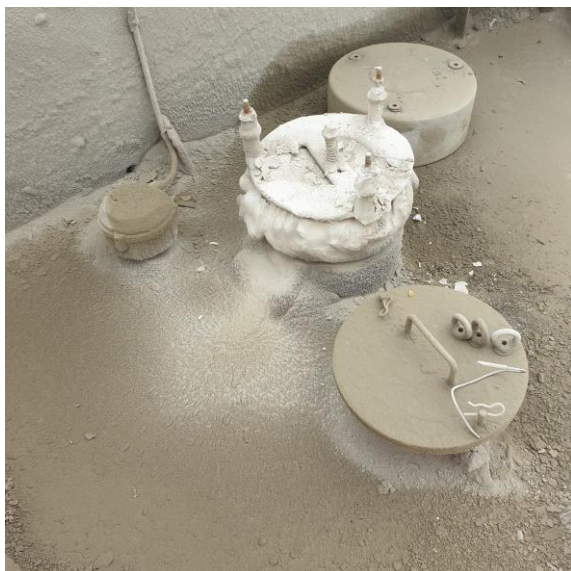
Blocked PRD – clearly in breach of permit condition but recorded as “OK”
