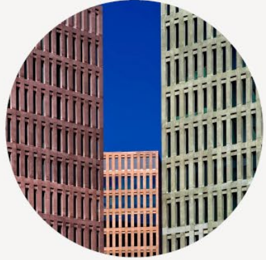
Building Circularity Design for Disassembly to reuse the building (blocks) over time
