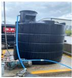
The team at Cemex's Springetts Asphalt plant in Stoke on Trent have recently made some Health and Safety improvements at the plant. The dust suppression system has been upgraded with new spay heads, a bigger water tank and a larger pump.
