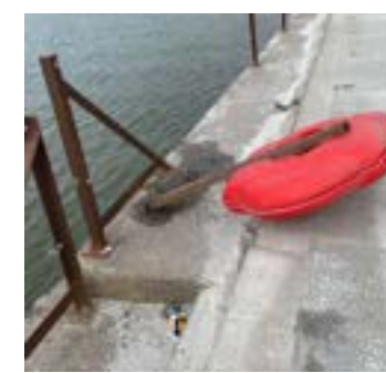
Lifebuoy post bent by rope
