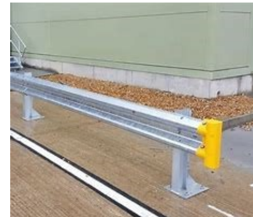
Typical Armco barrier end cap
