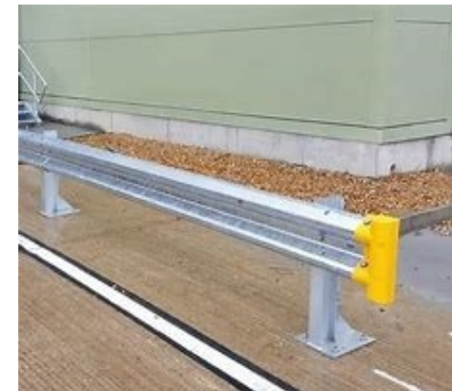
Typical Armco barrier end cap
