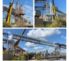
The team at Angerstein Wharf, close to the Thames barrier in London, has recently completed phase two of a major project to replace the Ship to Shore conveyor, which offloads sand and gravel from ships, into the plant.
