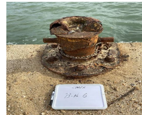
The failed bollard in 2020
